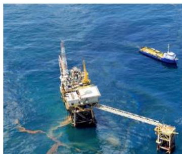
Oil platform leaks
